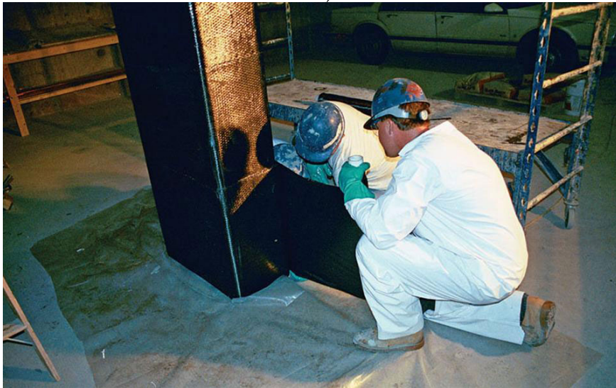
Figure 7. 1: Application of reinforced fabric wrapping on RC column; (a) application of first layer of reinforcement; (b) application of second layer of reinforcement, (ReLuis 2011)
