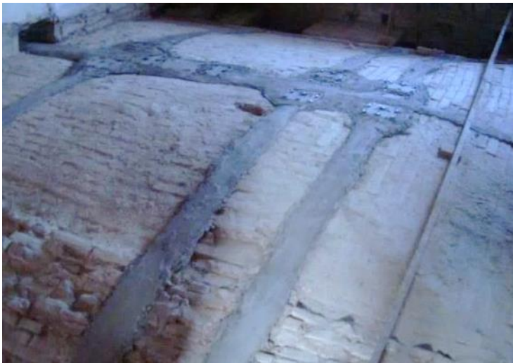
Figure 2.27 Extrados of the vault after the intervention [46]
