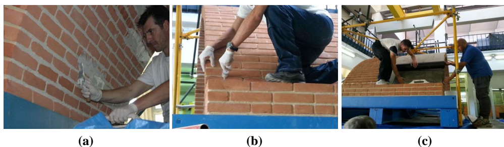
Figure 4.5 Resume of the retrofit process: (a) Repointing of the cracked joints at the intrados; (b) Grout injections at the extrados; (c) Grid installing layer at the extrados.
