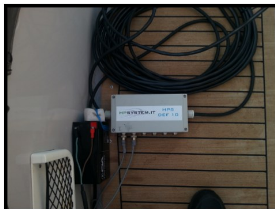
Figure 26: data acquired hardware
