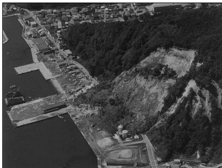
Figure 1.5. Okushiri-port Slide induced by the Hokkaido-Nansei-oki Earthquake (after Yamagishi, 2000)
