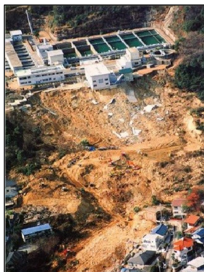
Figure 1.7. View of the Nikawa landslide (after Sassa et al. 1996).
