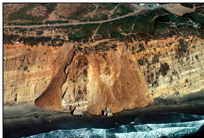
Figure 1.4. A huge landslide triggered along the coast.
