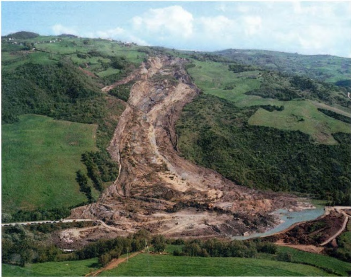
Figure 2.15. Main body of the 12th April 1996 Covatta Landslides.
