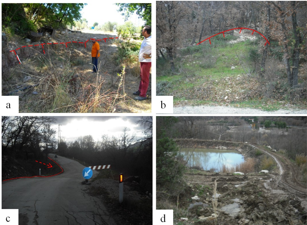
Figure 5.1. Main features of Roccavivara earthslide: a) and b) main scarp; c) body of the landslide, which affected the roadway; d) artificial pond located at the toe of the slide.
