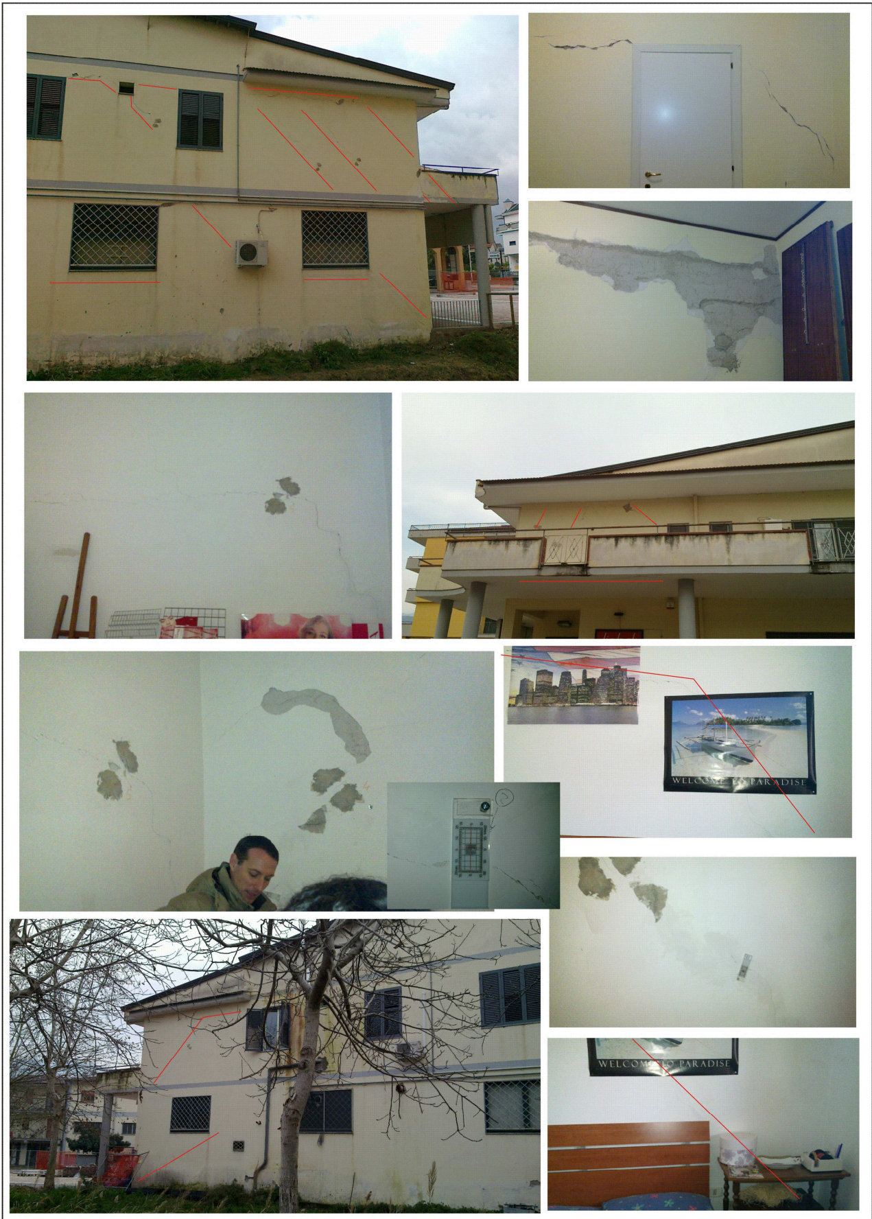
Figure 6.74: Forensic analysis of the building n°2
