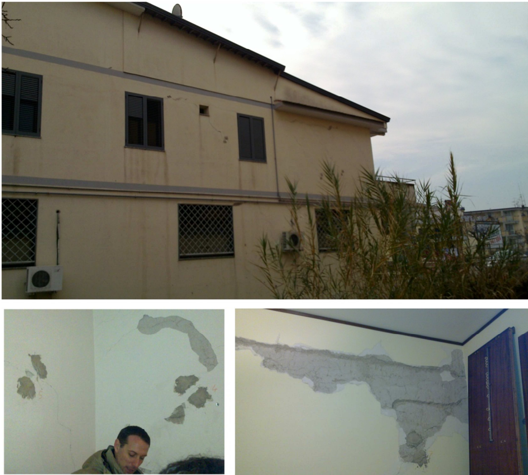
Figure 3.7: example of cracks monitoring in Telese Terme
