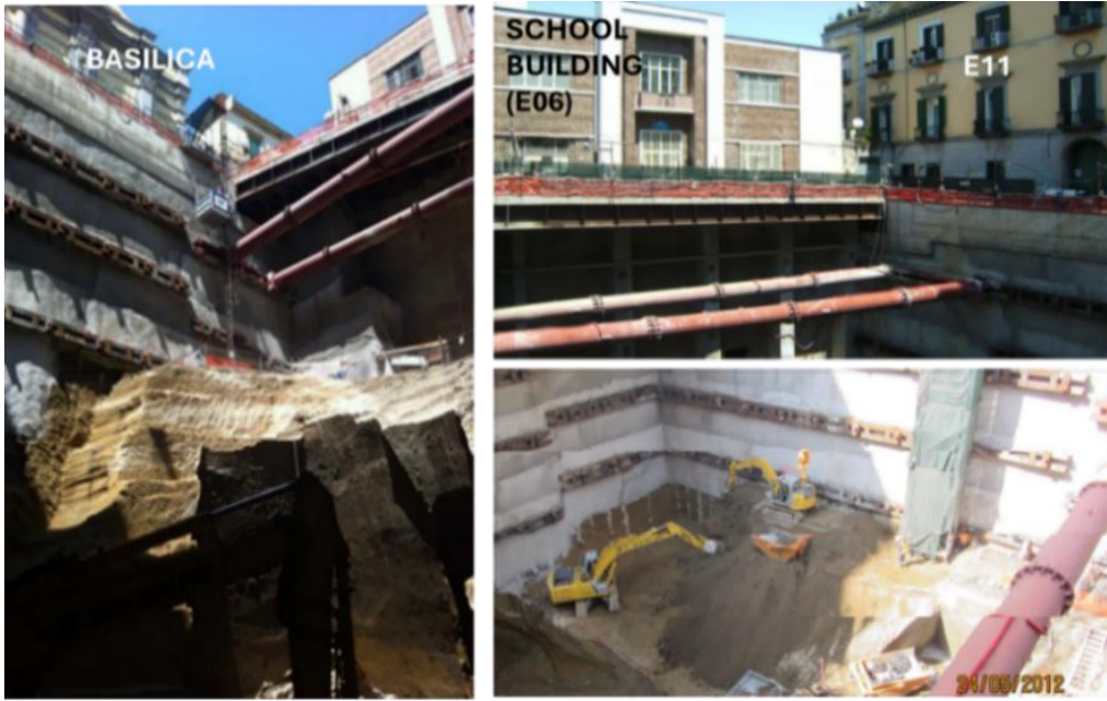
Figure 38. Pictures taken during excavation.
