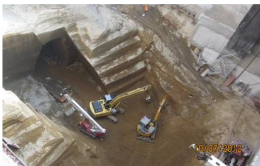
Figure 39. Above: plan view of the station with the indication of anthropic cavities, and below: pictures of the cavities interfering with the work.
