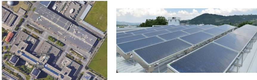
Figure 40. Existing Geneva solar field.
