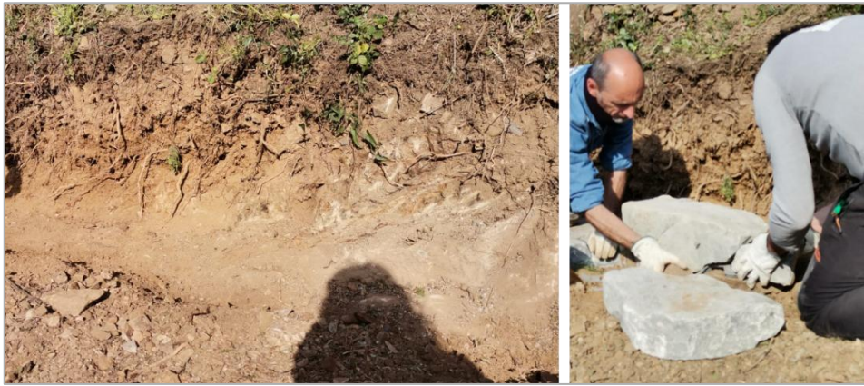
Figure 3.17 - Excavation operations placement of rock blocks for the wall's foundation on the weathered bedrock.
