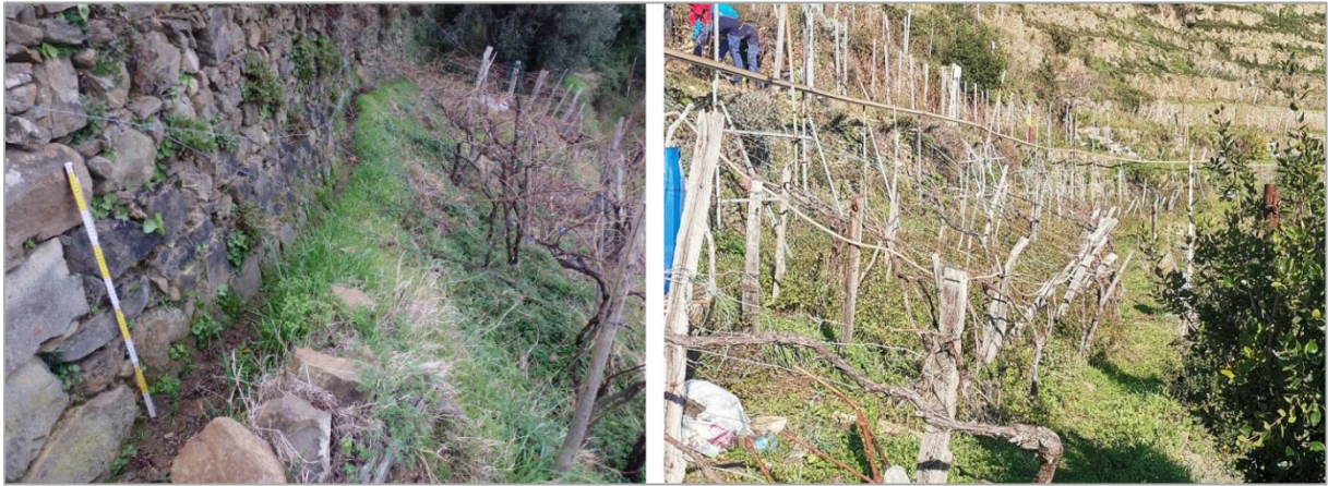
Figure 2.11 - On the left, a drainage channel at the base of a wall is illustrated; on the right, the sub-horizontal inclination of a terrace is visible (from Bernini et al., 2021).
