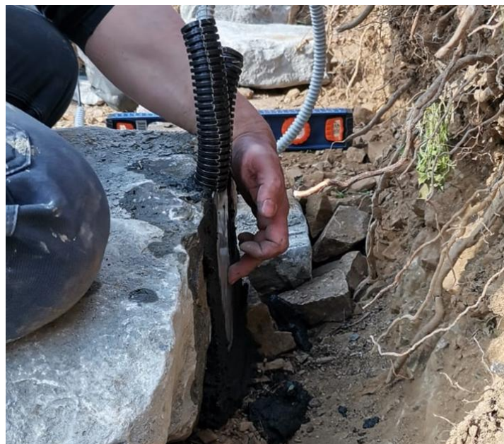
Figure 3.18 – Installation of pressure cells behind the wall.
