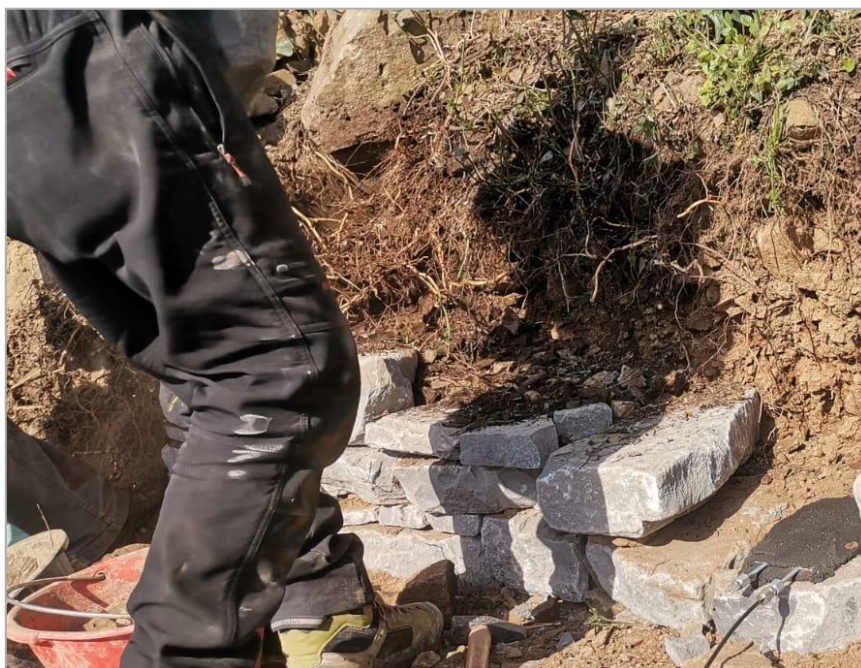
Figure 3.19 - Detail of the backfill material used during wall construction.
