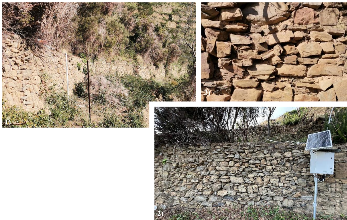
Figure 2.17 – Characteristics of the dry-stone wall terraced system at Site 846: 1) lateral view of the abandoned terraced area covered by spontaneous vegetation; 2) detail of the sandstone blocks constituting the wall; 3) monitored terrace section.
