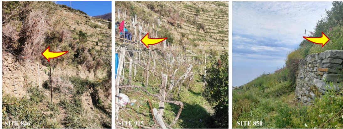
Figure 3.11 - The yellow arrow indicates the area upstream of the retaining wall, where the sensors were installed for each experimental monitoring site.
