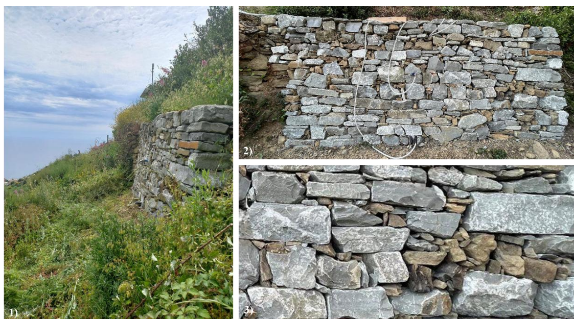
Figure 2.19 - Characteristics of the dry-stone wall terraced system at Site 850: 1) Lateral view of the terrace; 2) Frontal view of the new masonry rebuilt using traditional building methods; 3) Details of the different sandstone-marly limestone blocks forming the wall.
