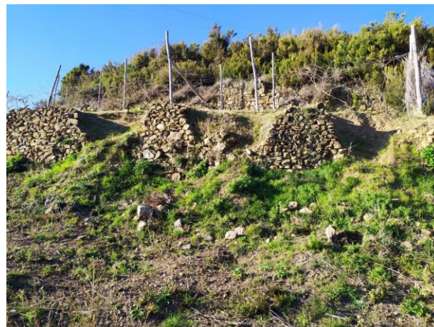
Figure 2.10 - Examples of wall collapses in the study area, developing along the line of maximum slope (from Bernini et al., 2021).
