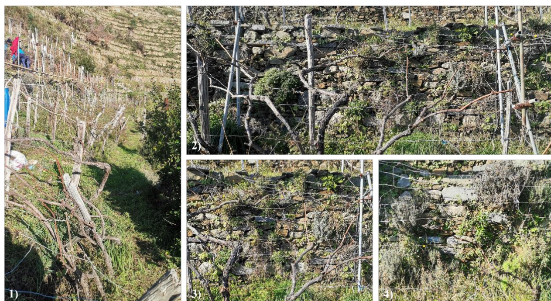
Figure 2.18 - Characteristics of the dry-stone wall terraced system at Site 915: 1) View of the terraced vineyard; 2) Details of the dry-stone wall structure and of the “ pergola ” type vineyard cultivation.
